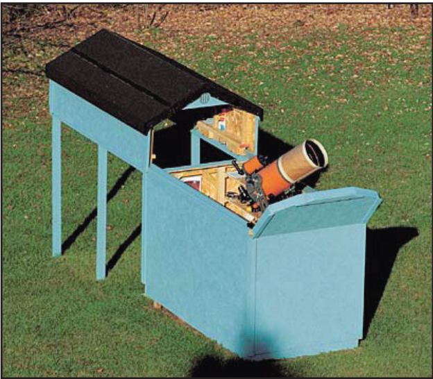
Fig 2: Model of a roll-off roof observatory
